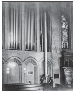
Robert L. Meunier (left) and Fred H. Meunier installing CCCC of the 32ft Open Diapason at Saint John's Cathedral, Denver, March 1938
