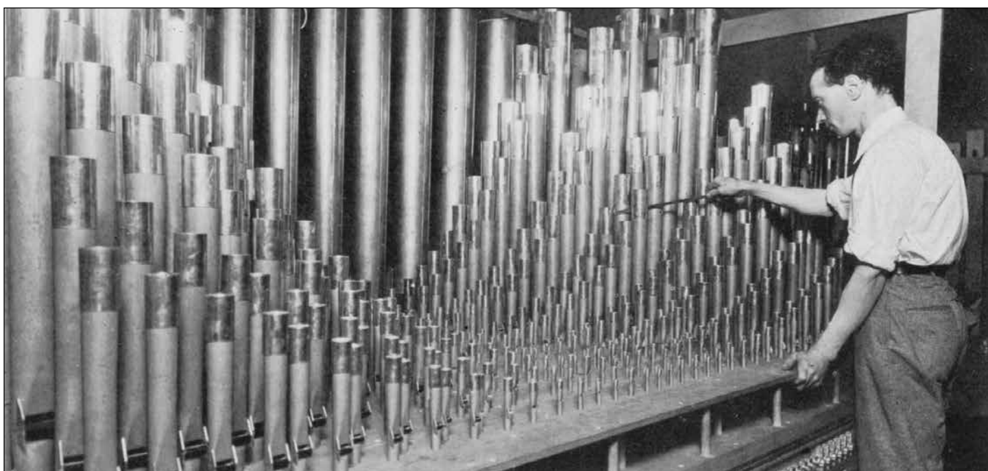
H. Vincent Willis tuning the 7-rank double-languid Stentor Mixture on 35" pressure made with double languids and flared 4 notes wider at the top than at the mouth and by far the most powerful and brilliant Mixture ever made. CREDIT: Under the Sassafrass Tree , Midmer-Losh, 1930
